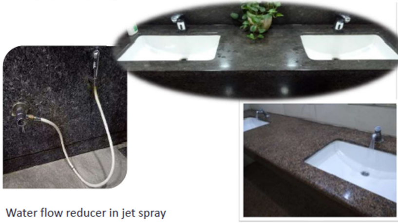
Water sensor taps in wash basins
